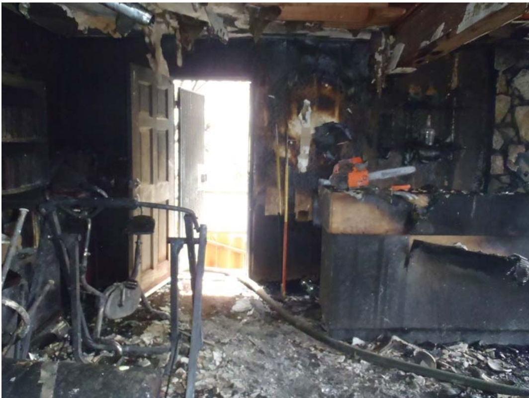
In the fire room looking out towards the door on the Bravo side, this is the door that Engine 11 and Battalion 9 made entry from.
