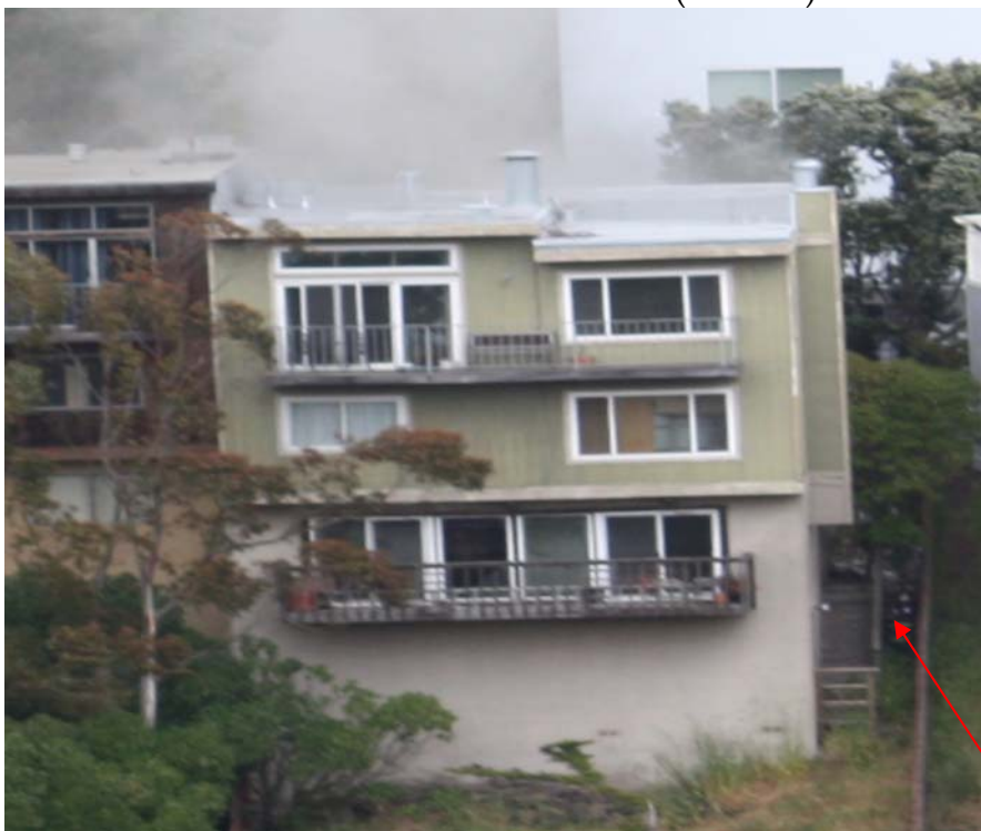
10:57:11 First picture showing conditions from the rear of the building. Note Battalion 9 coming down the hill side on the Bravo side. Noticing a metal gate on the door to Sublevel 1, Battalion 9 requests a forcible entry tool. (6565)
