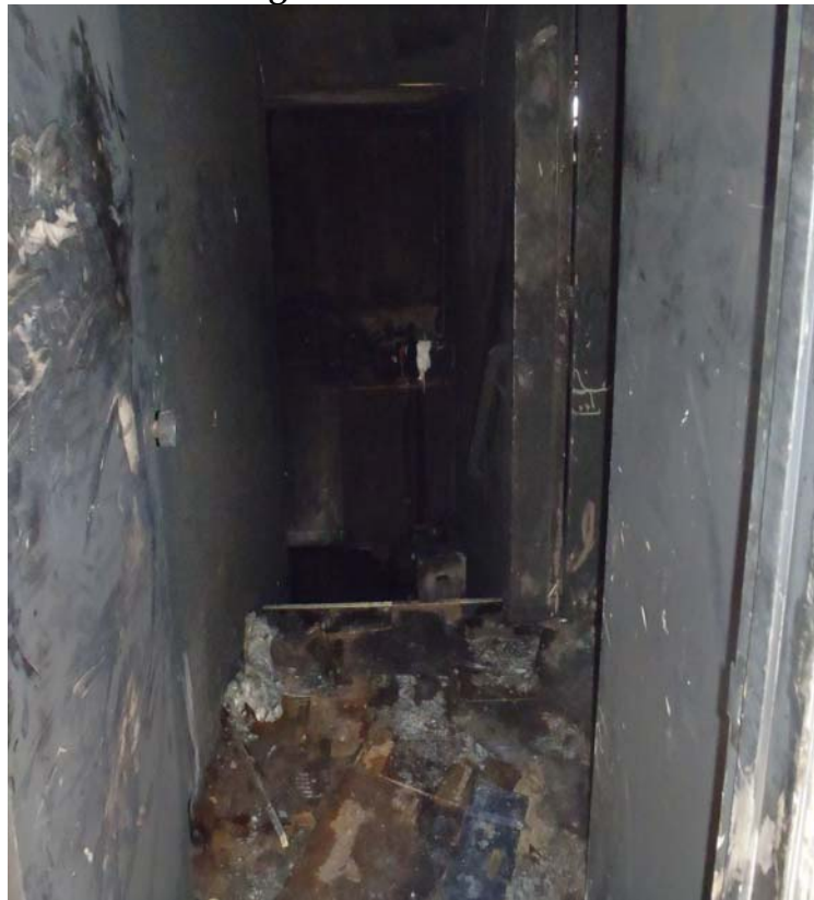
Top of stairs leading down to fire room, note amount of carbon material deposited on the surfaces
