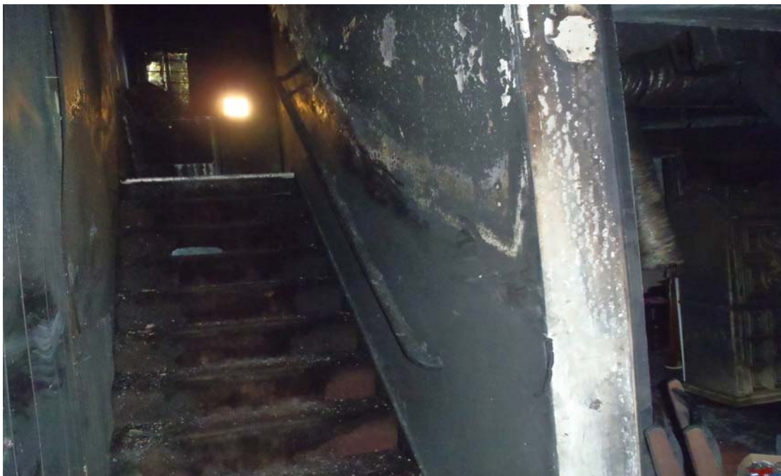
Looking up the stairs from the fire room, note the heat damage on the walls
