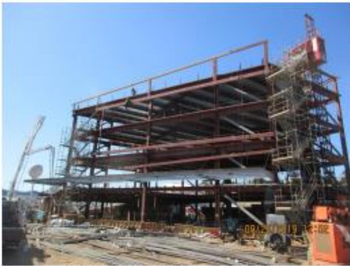
Erection of Steel Canopy – September 20, 2019
