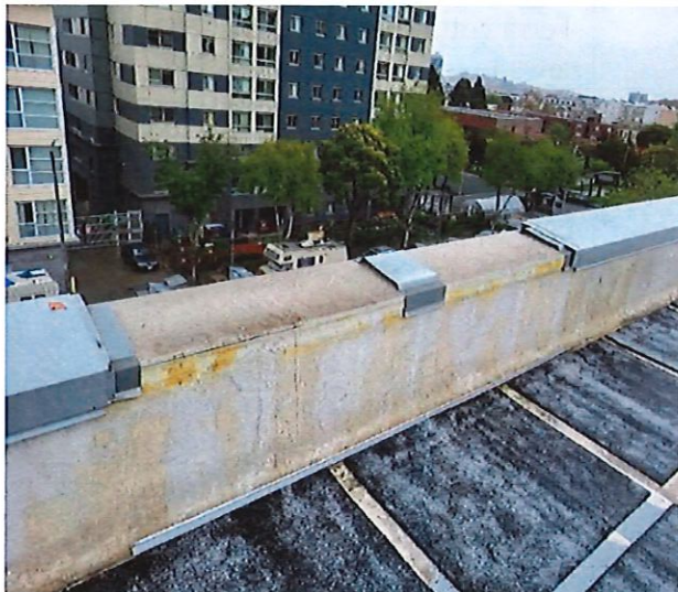
Roof of Station 5 where flashing blew off
