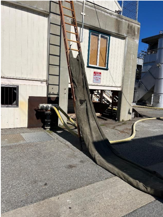
Salvage cover used as a chute
