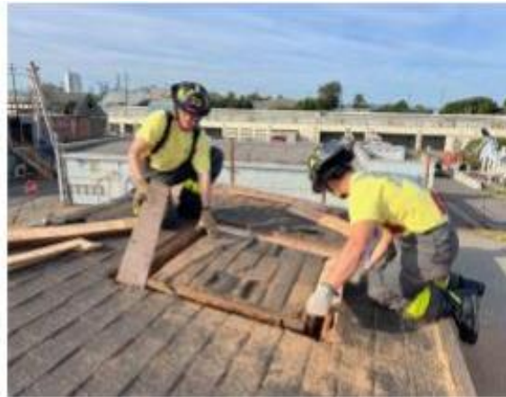
Reframing the Peaked Roof Prop
