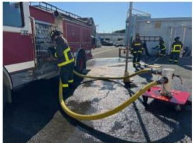
Low Pressure Hydrant
