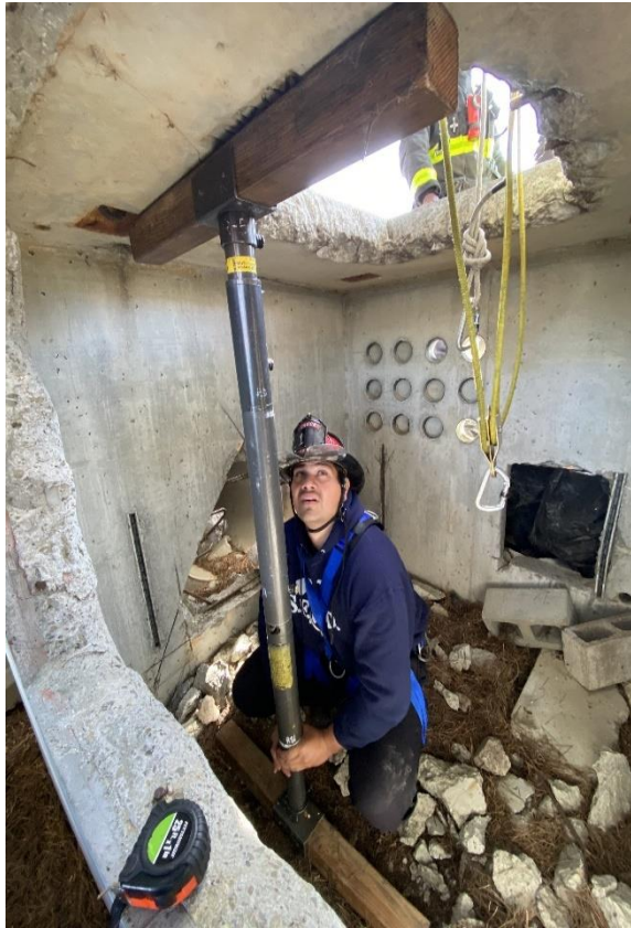
Making the area safe by stabilizing a weak ceiling with Paratech shores.
