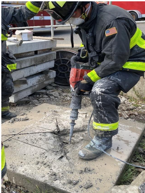
FF with electric concrete breaker/chipper.
