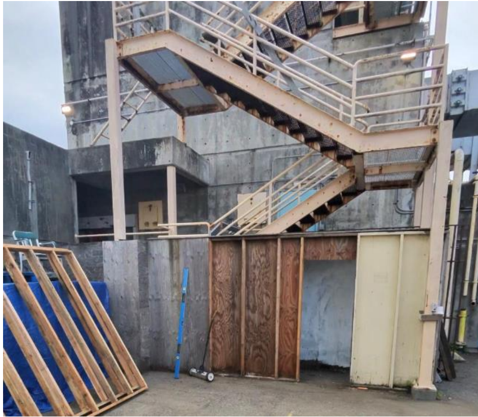
Burn Room Construction at TI
