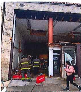
Breaching and Breaking, 1523 Franklin
