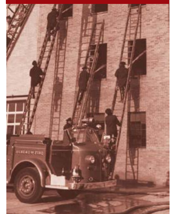
Photo Courtesy of the Philadelphia Fire Department
