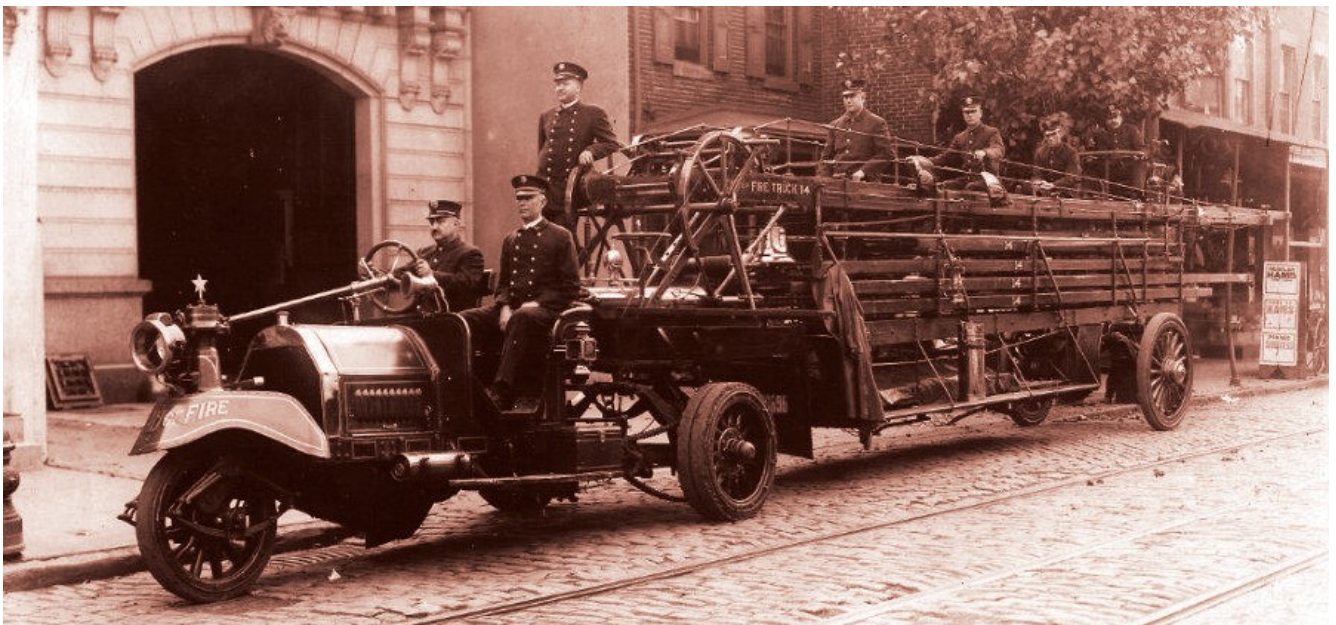
Photo Courtesy of the Philadelphia Fire Department
